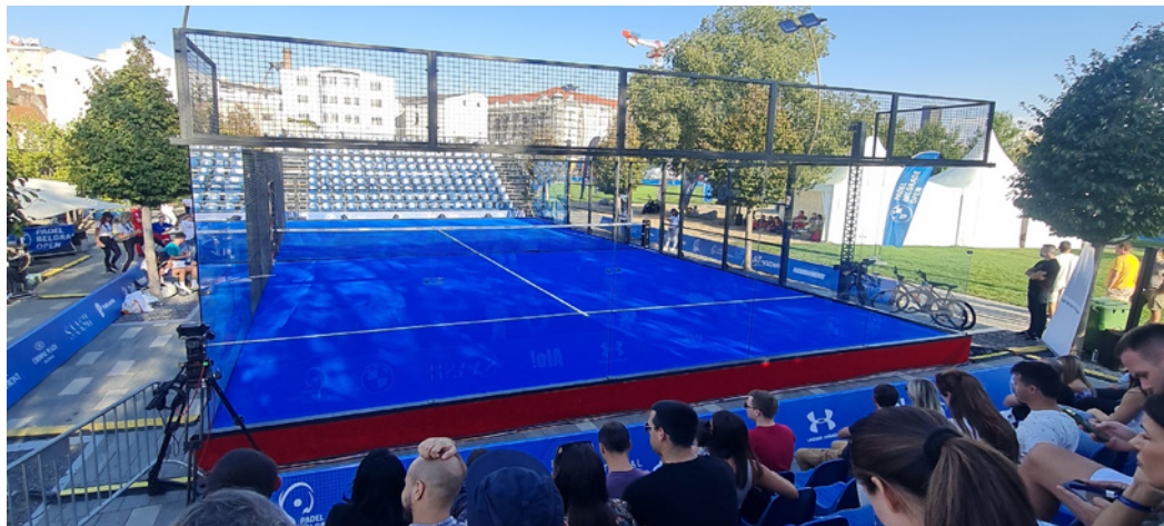
Platform and Premier model field installed for the Belgrade Open, Serbia, 2023
